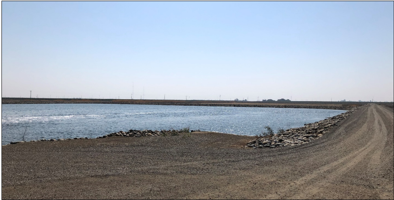
Photo 3-2. Existing WWTF Ponds
